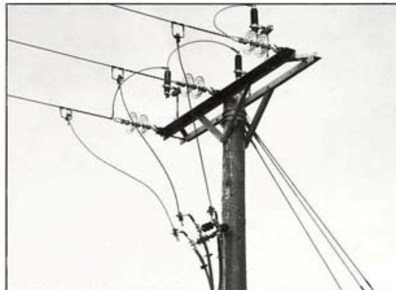
HEAT SHRINK CABLE TERMINATION WHERE BI-METAL LUGS AND SPLICES MAY BE USED.
